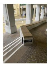
The 2 ramps are 6.5m long with a gradient of 1:12, and 940mm wide at the narrowest point. There are currently no handrails on the ramps.
