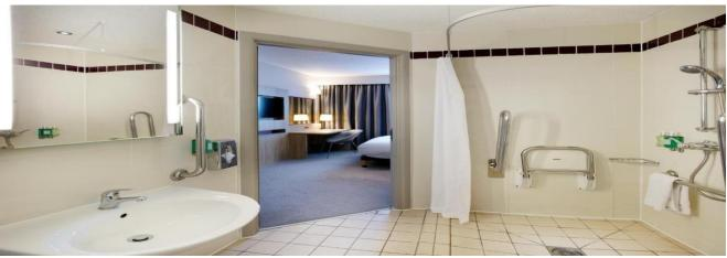
The clear door opening width of the bathroom door is 36" (91cm).
