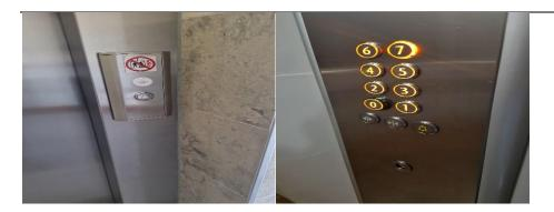
Top floor lift buttons are 54.5" max height and the lift call button is 44.5"
